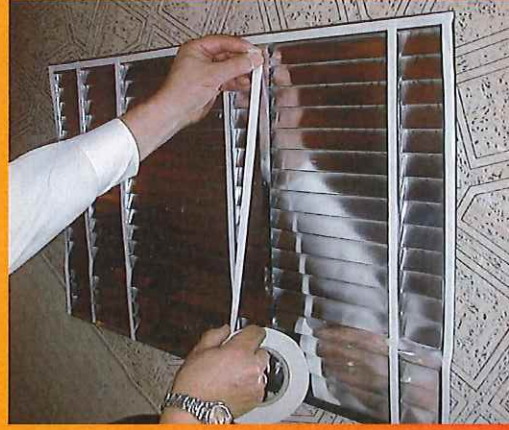
Apply Double Sided Tape to Sempatherm Panels
