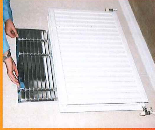
Fit Sempatherm Panels in place
