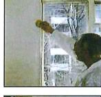
Using SEMPATAP EDGING TAPE to achieve a neat finish on all outward facing corners, window reveals, window heads, etc. locate over the corner of the SEMPATAP and smooth out.
