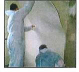
SEMPATAP is applied foam side to the wall. Cut SEMPATAP to required length then roll up with foam side facing out. Apply SEMPATAP to wet adhesive, roll out and smooth with light level hand pressure. Firm up using SEMPATAP SPATULA.
