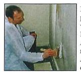
Remove any wallpaper and prepare the walls as though you were going to decorate. Apply a liberal coat of SEMPATAP ADHESIVE to the wall using the notched SEMPATAP ADHESIVE SPREADER, brush or roller.
