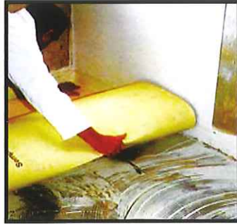
Roll out SEMPAFLOOR insulation
