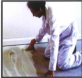
Apply SEMPATAP ADHESIVE to floor surface
