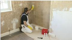
**Mould growth** on walls and ceilings must be treated with a MGC Mould Eradication Kit in accordance with MGC Mould Eradication Instructions as follows.
